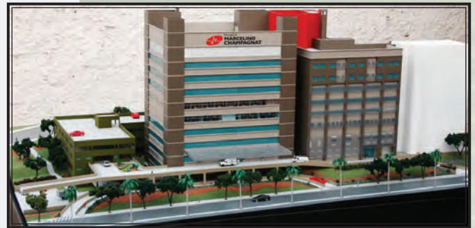
This photo depicts a model of the Hospital Marcelino Champagnat (HMC), Curitiba's "gold standard" hospital. HMC is the only private hospital in a system that owns four other large public hospitals. HCM was built to cater exclusively to private patients, but the group was fascinated to learn that the facility's profits are used to subsidize the four other not-for-profit hospitals in the system.
