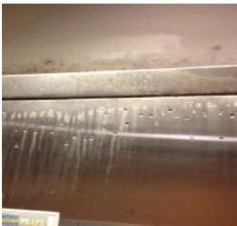
Figure 3. Visible condensation on cold room door handle.
