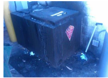
Kitchen grease storage with spillage
