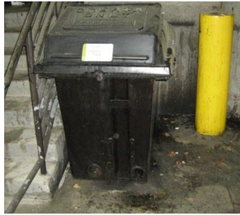
No secondary containers for some primary containers
